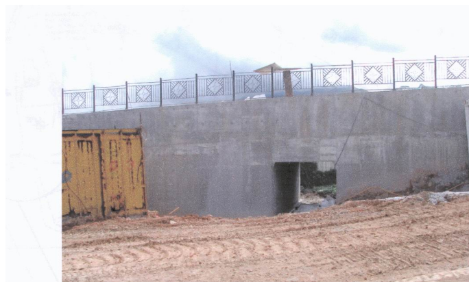
Photo taken on: 22 July 2003 (Front Elevation of the Ramp Structure)
